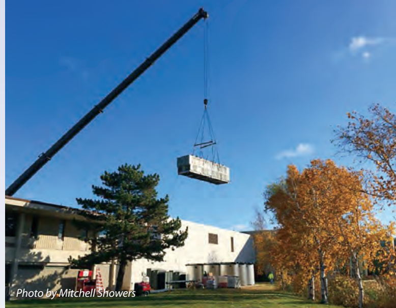
A new large chiller unit is lifted over the Science Building at UW-Fond du Lac in the fall of 2015 and placed near the University Center. This was just one component of a year-long energy improvement project which will reduce the university's energy costs and provide educational opportunities.
