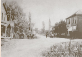
Building at left (1908) is currently The Granary.
