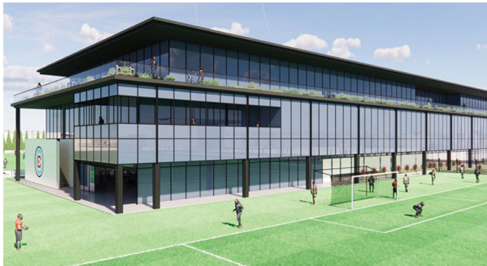
The Chicago Fire and City of Chicago have proposed building a training facility on Chicago Housing Authority land in the Roosevelt Square area on the Near West Side.
